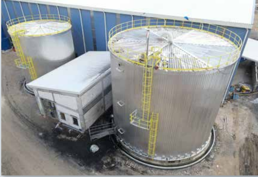
■ Raw Water, Demineralized Water Tanks
