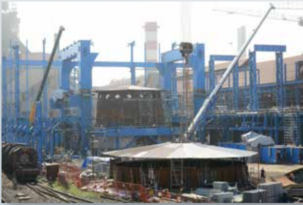
■ Blast Furnace Preassembly and Erection View
