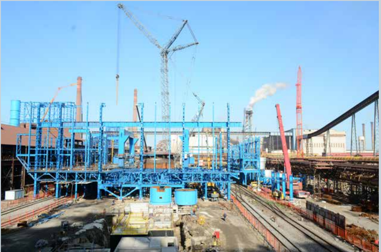
South Slag Granulation Plant and INBA Structure and Casthouse Steel Structure South View
