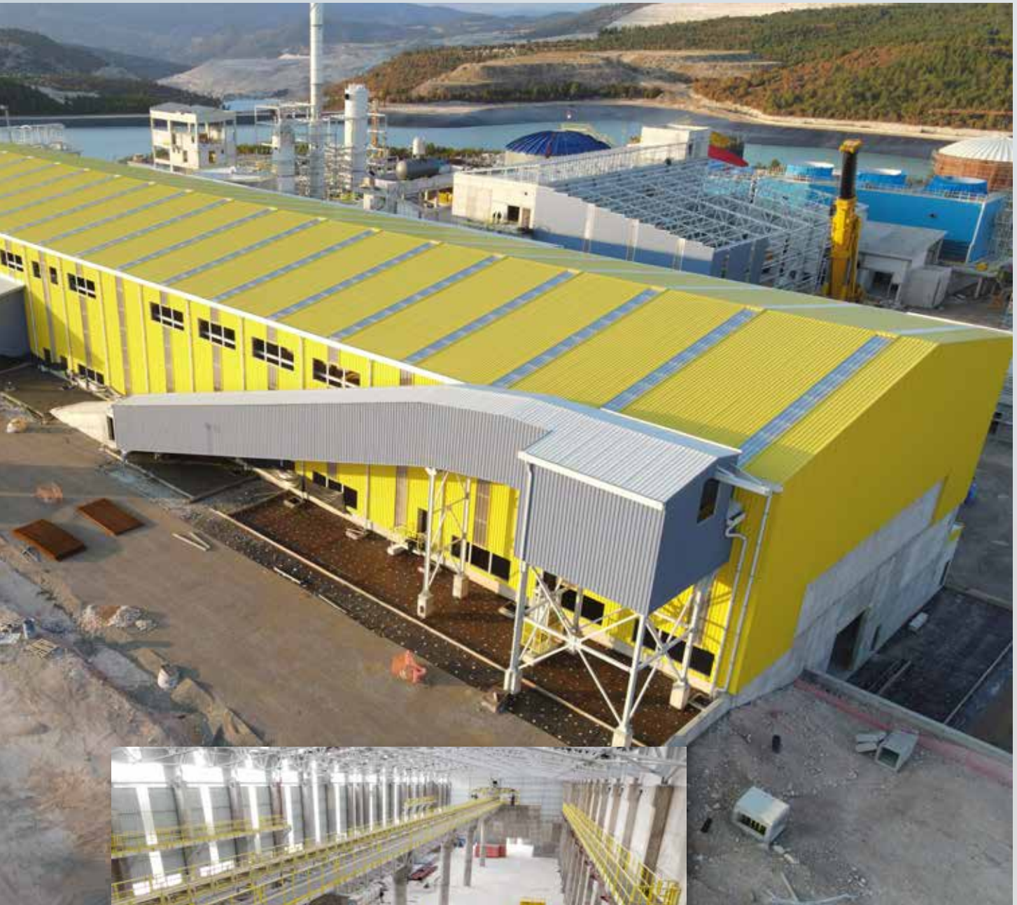
Sulphur Storage Building ■
