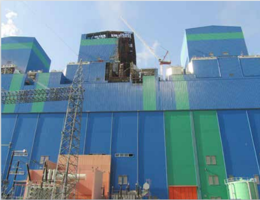
■ North Facade Dismantling Works
