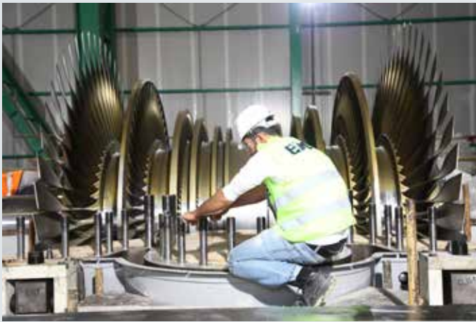
■ Steam Turbine Erection
