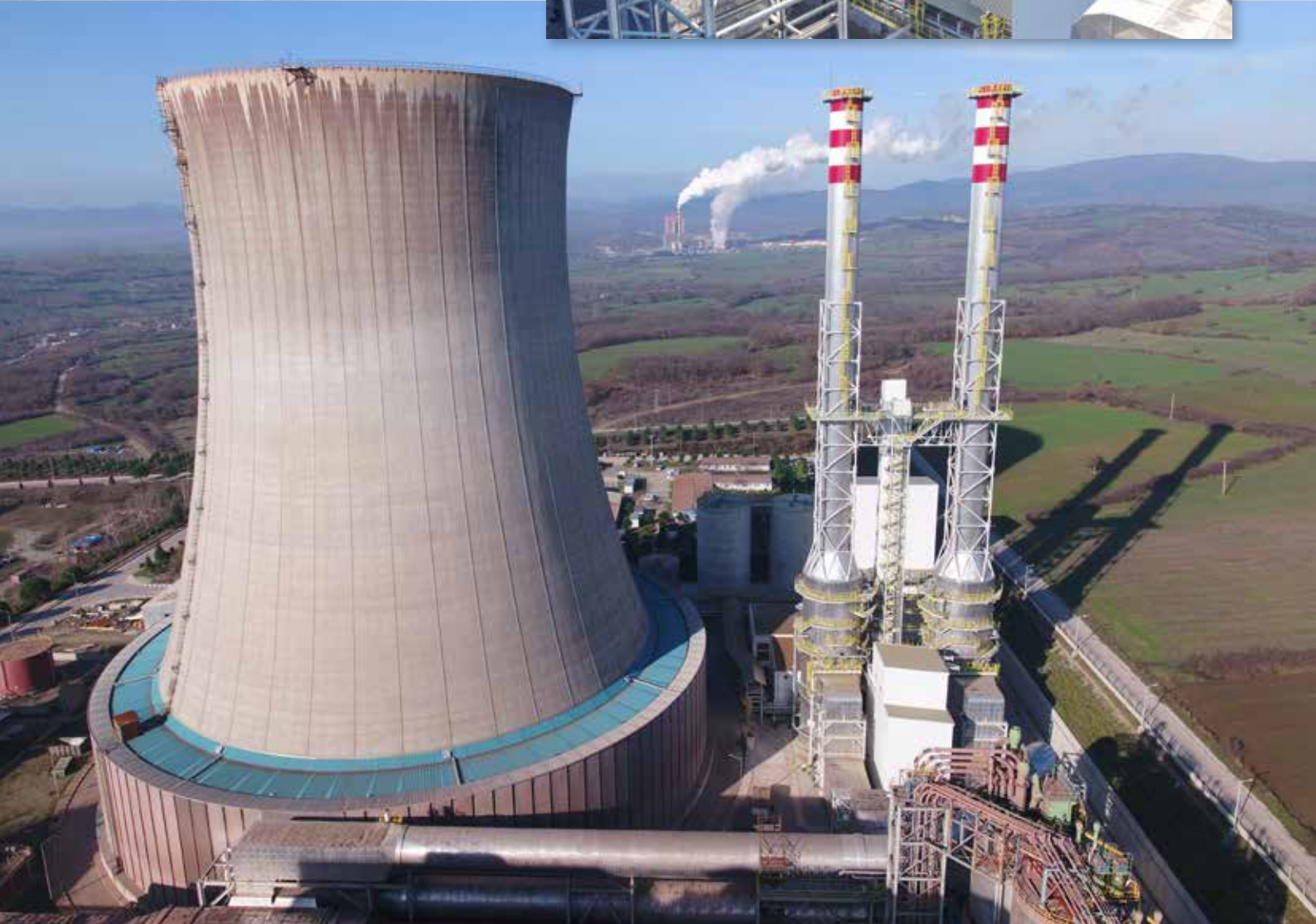
■ General View of Site
