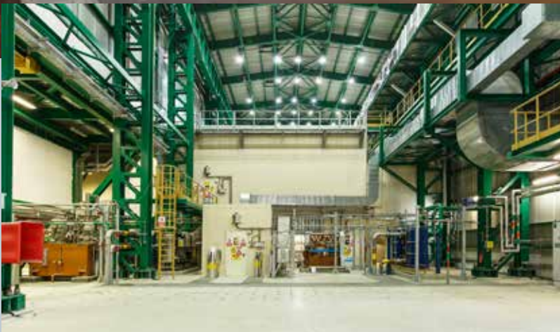
■ Gas Turbine Hall
