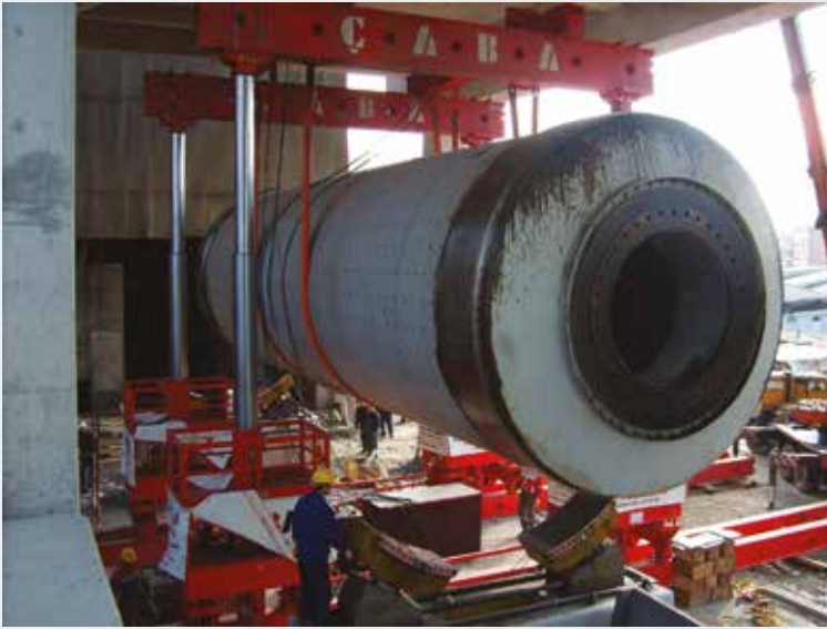
■ Erection of Ball Mill
