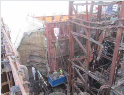
■ Cladding Dismantling Works
