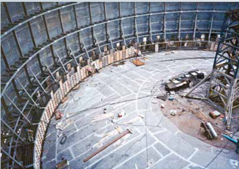
■ Construction Works at Floating Piston
