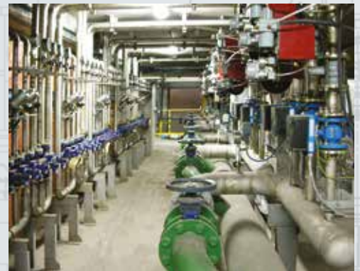
■ Valve Control Room
