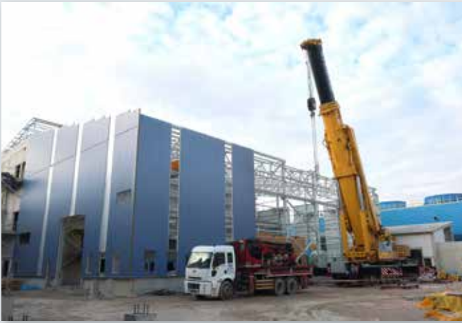
■ Electrical Building, Turbine-Generator Building
