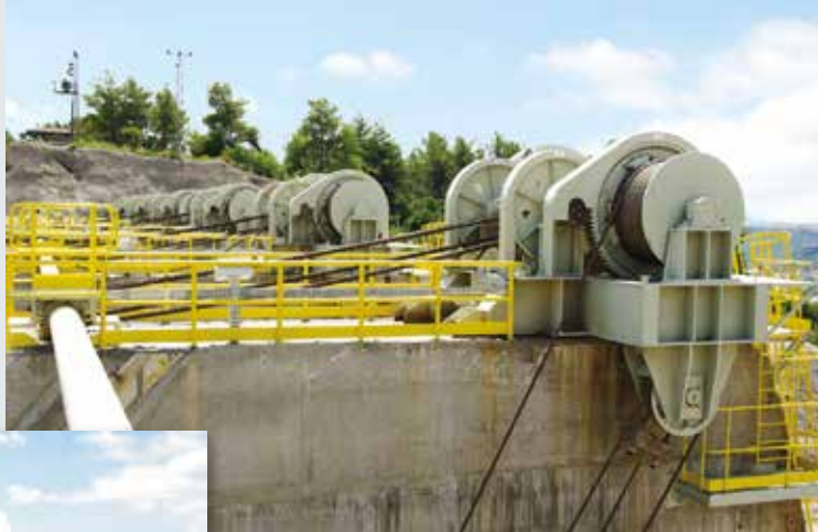
■ Radial Gates Operating Mechanism
