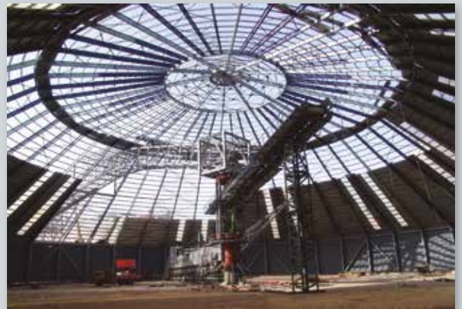
■ Erection Works at Circular Storage Area
