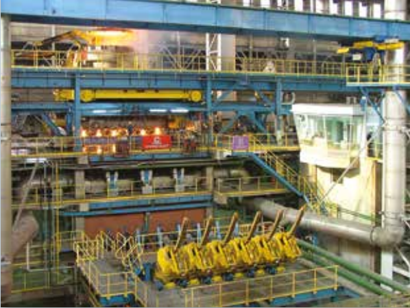
■ General View of Plant
