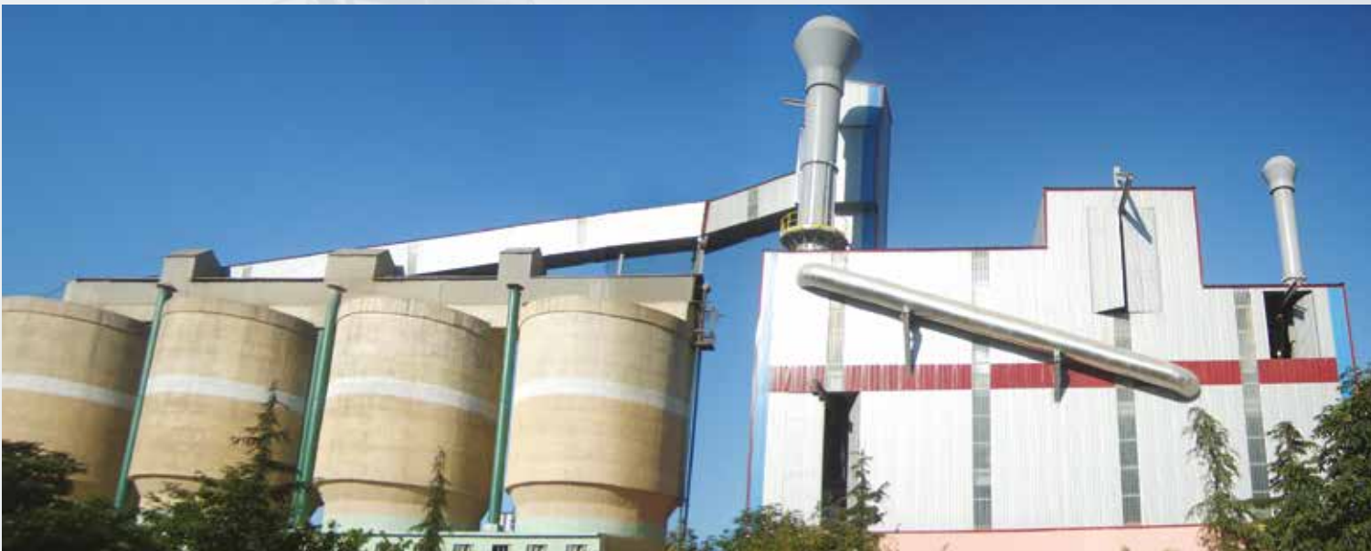
■ Cement Silos and Cement Grinding Plant
