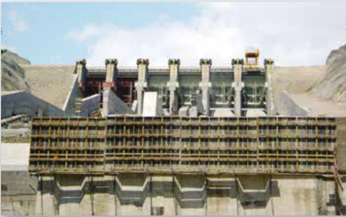
General View of Spillway and Radial Gates from Outlet
