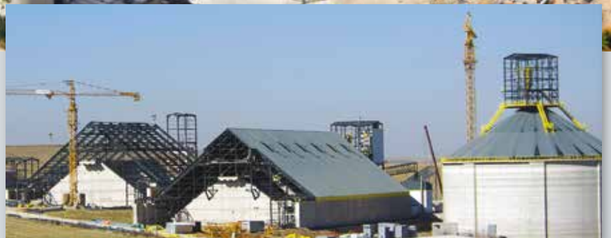
■ Coal and Additives Storage Buildings and Clinker Silo
