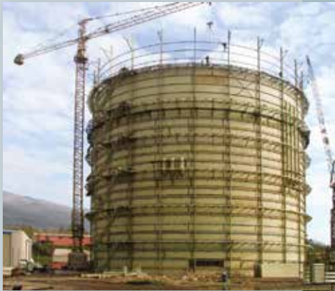
■ Construction Works at Outer Shell
