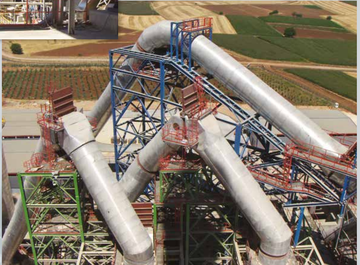
■ Raw Mill Gas Ducts
