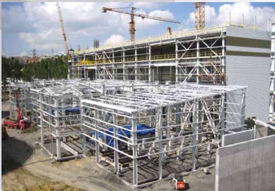
■ Gas Turbine & Generator Building
