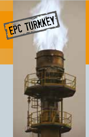
■ Blast Furnace Excess Gas Flare Stack
