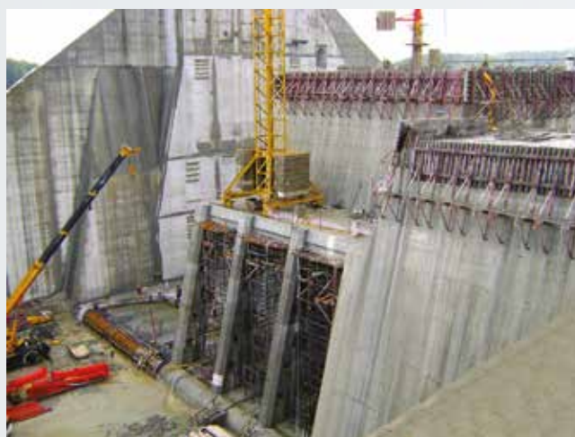
■ Construction Works at Water Intake Structure
