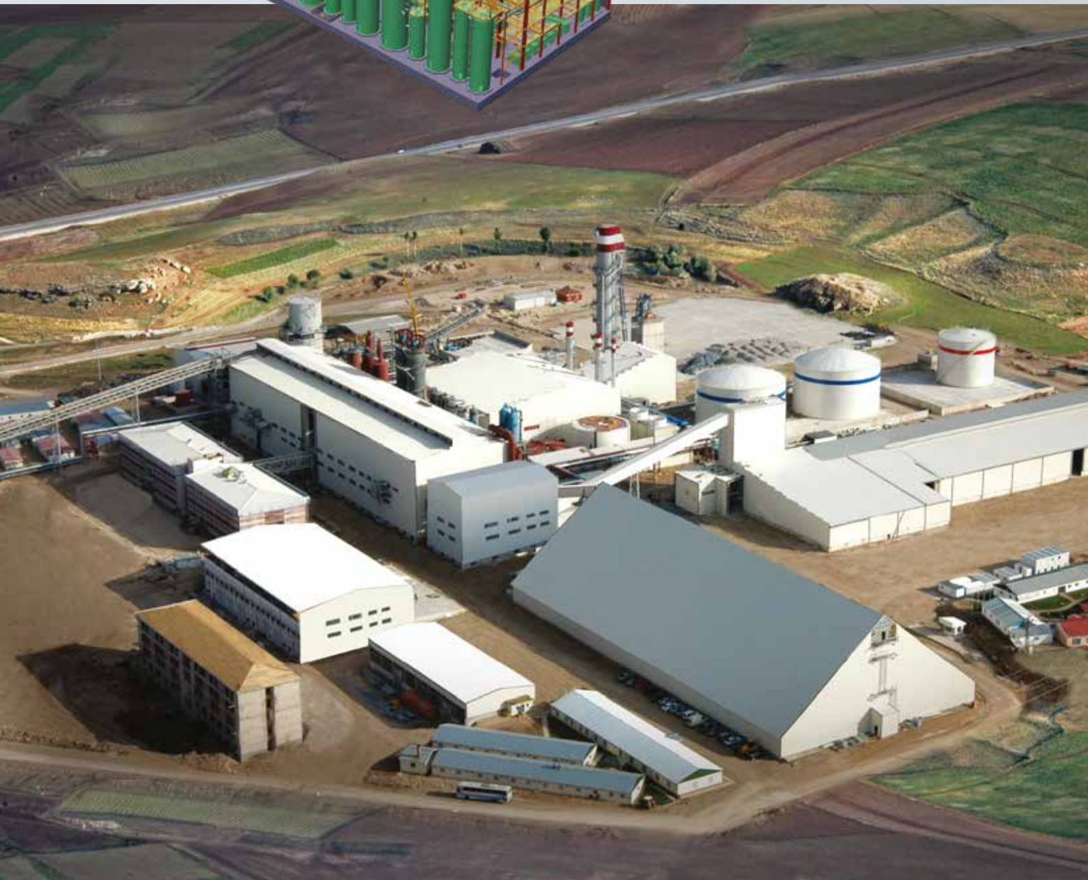
■ General View of 10,000 tons/day Sugar Beet Slicing Capacity Boğazlıyan Sugar Factory
