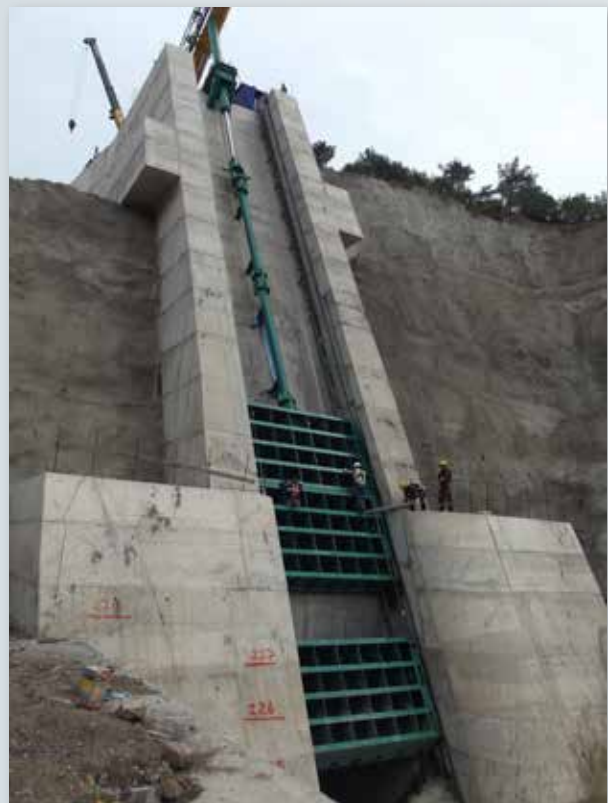
■ Sluiceway Inlet Gate
