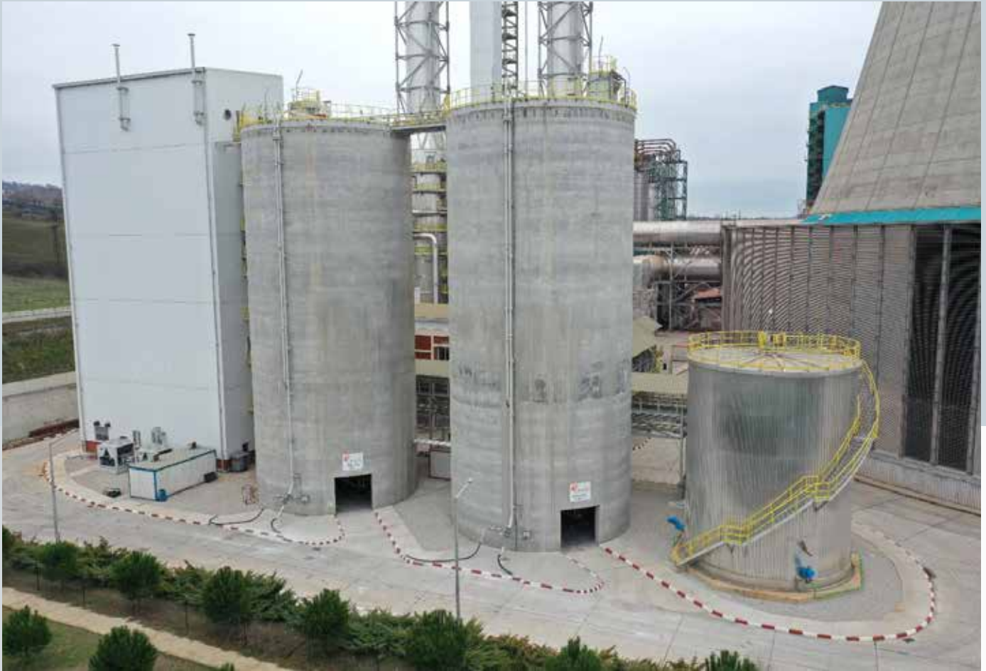
■ Limestone Storage Silos & Limestone Slurry Building & Emergency Storage Tank
