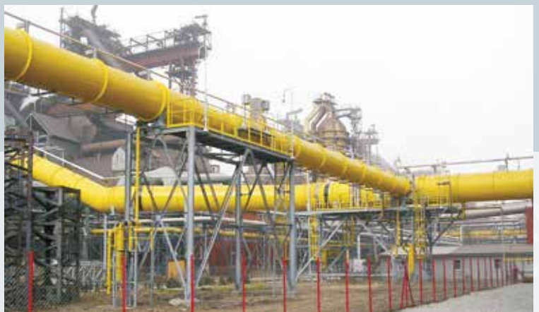
■ A View from Gas Duct
