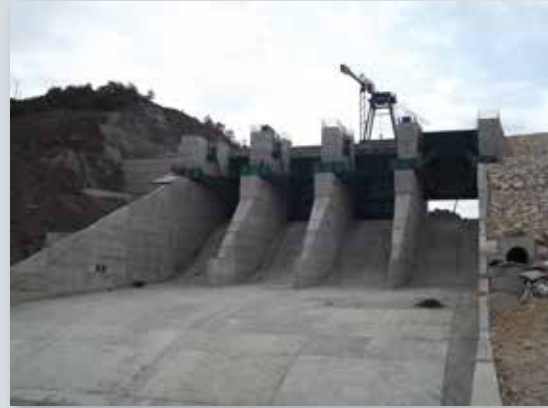
■ Radial Gates of Spillway Downstream Face
