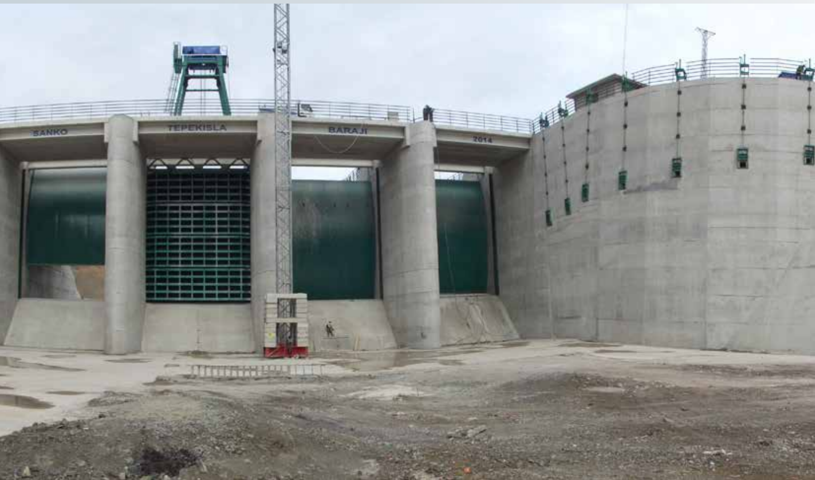
■ Radial Gates of Spillway and Fish Passage Gates, Upstream Face
