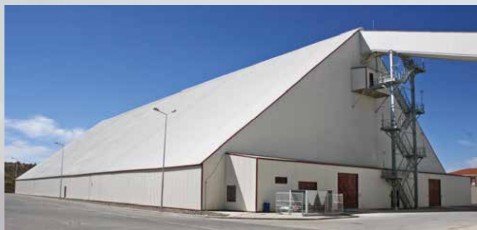
■ Sugar Silo (60,000 tons, 116.5 x 57.8 x 50 m)
