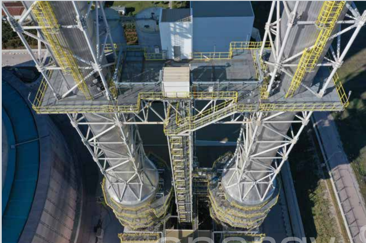
■ Wet Stack Steel Structure & +65.00 Level Platform
