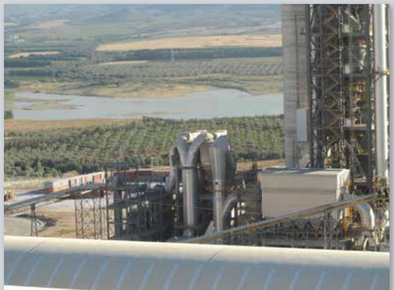
■ Raw Mill - Exhaust Gas Conditioning
