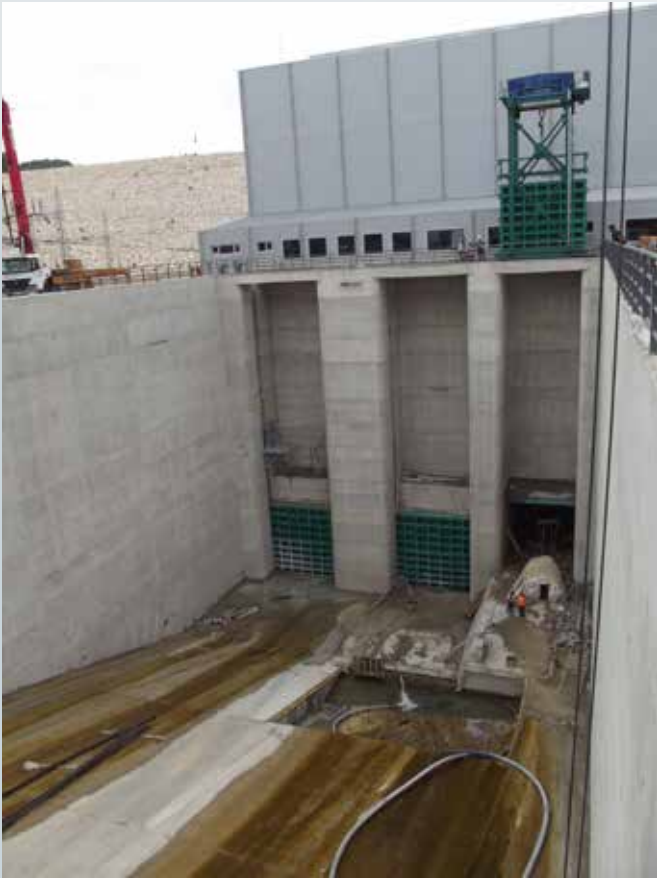
■ Downstream of Power House
