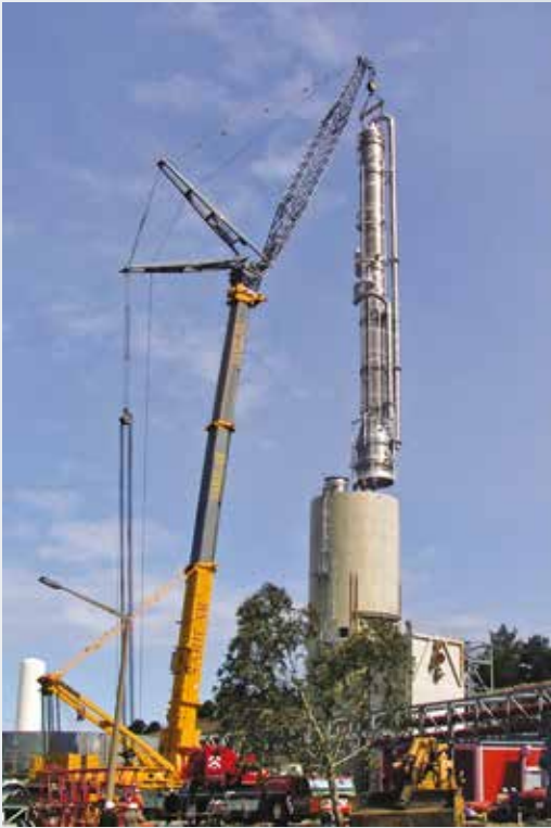
■ Erection of Cold Box
