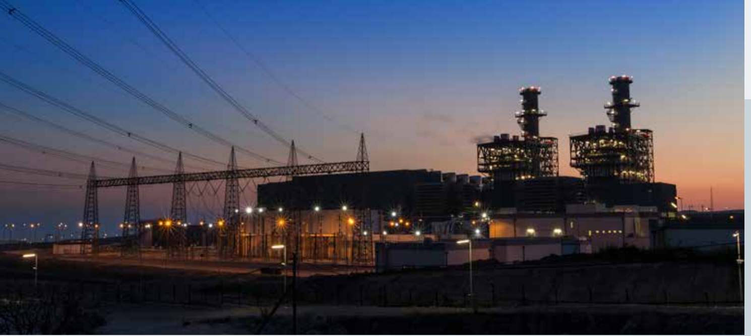
View of Switchyard ■
