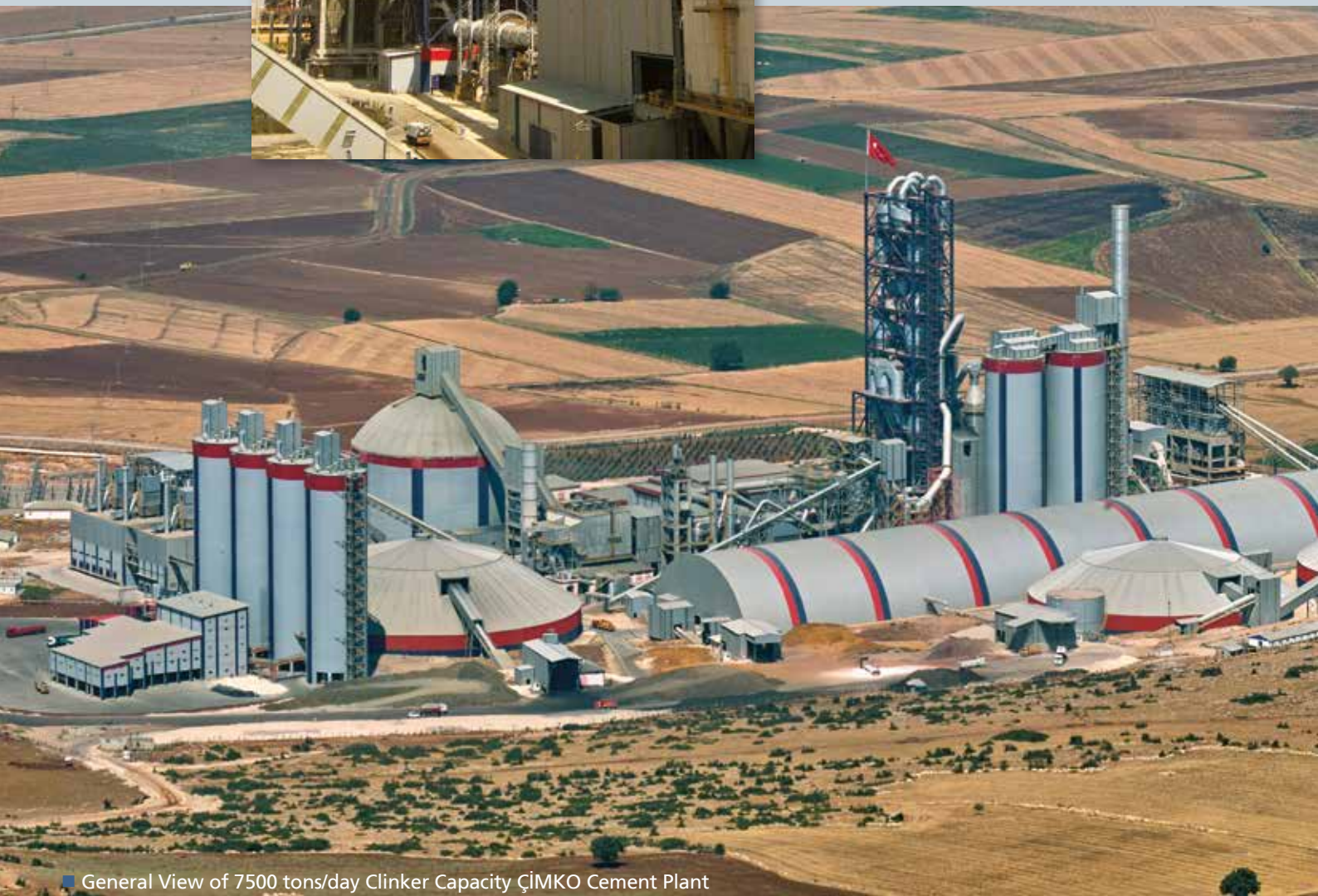
■ Circular Limestone and Longitudinal Shale Blending Bed
