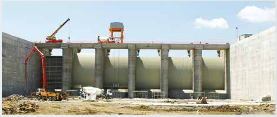
Spillway Intake Structure and Radial Gates
