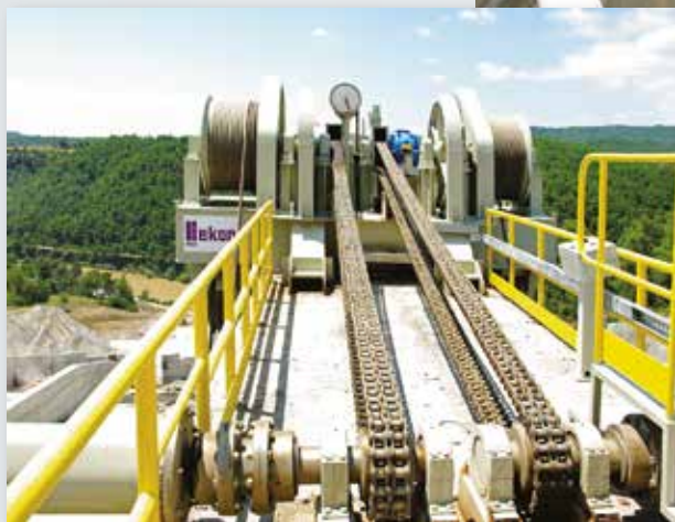
■ Radial Gates Operating Mechanism
