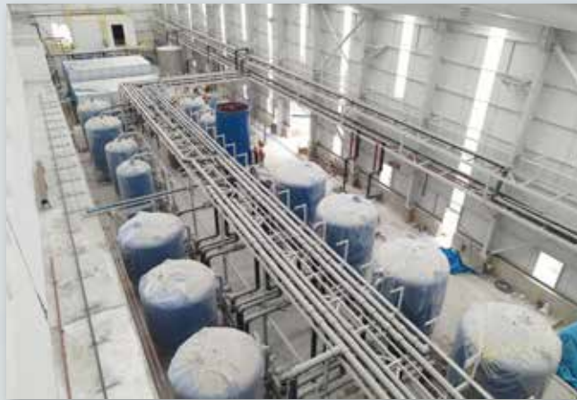
■ Demineralized Water Treatment Building
