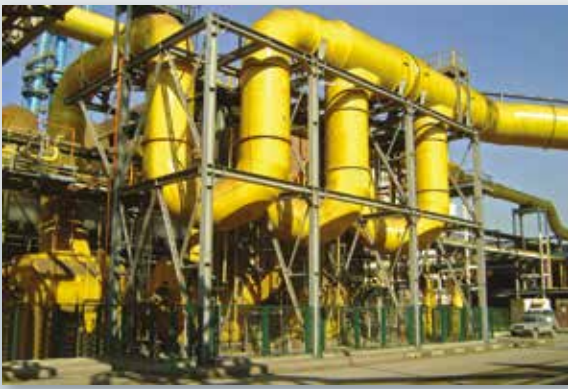
■ Gas Recovery Station
