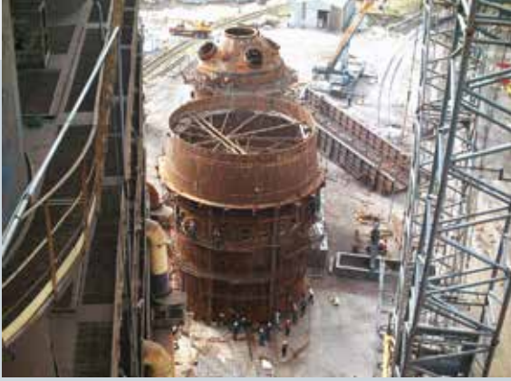
■ Site Manufacturing of Blast Furnace Body
