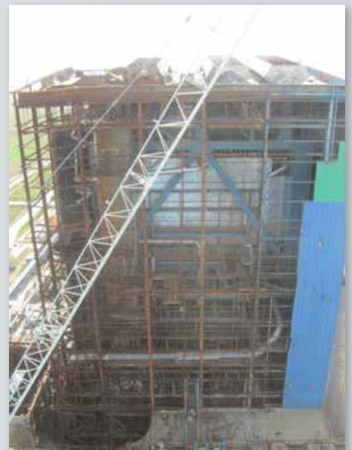
■ West Facade of the Damaged 2nd Unit
