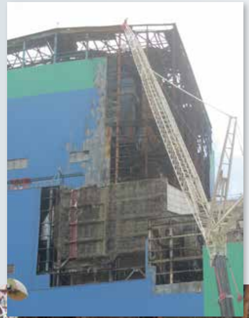
■ North West Facade Dismantling Works
