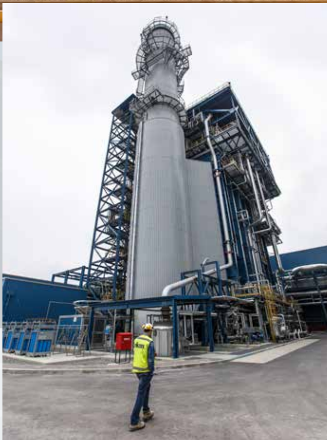
■ Heat Recovery Steam Generator
