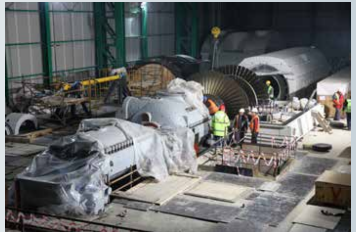
■ Steam Turbine Erection
