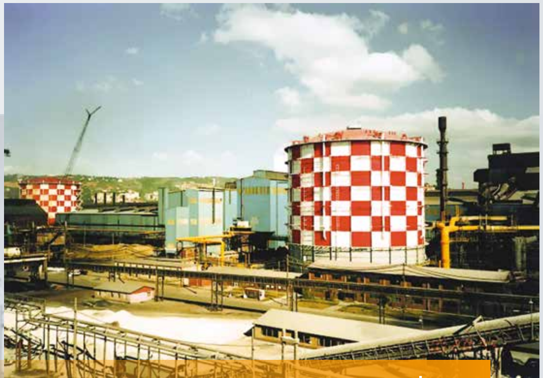
General View of the Plant ■
