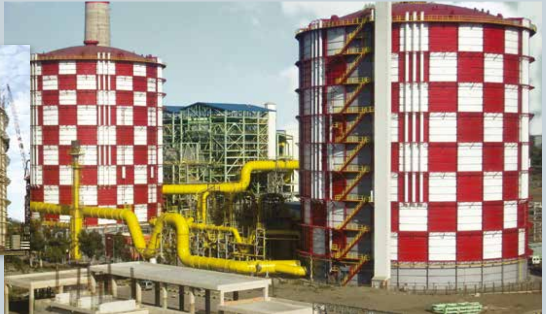
General View of the Plant ■
