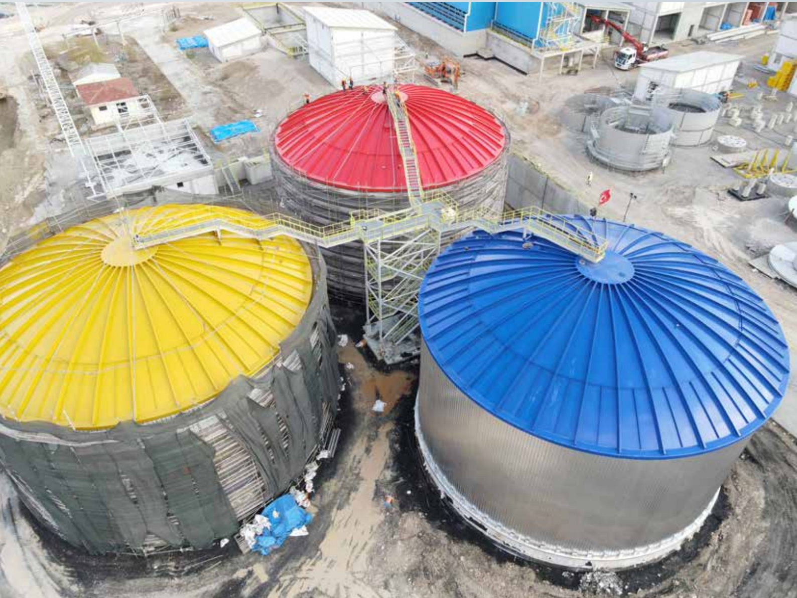
■ Acid Storage Tanks
