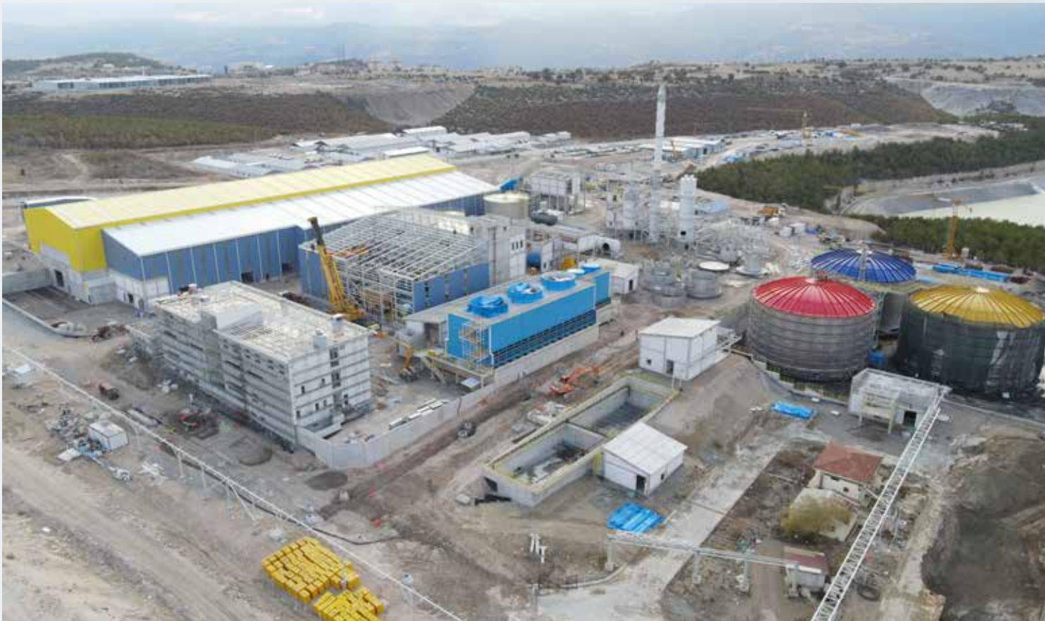
■ General View of Site
