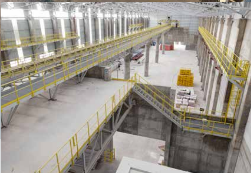
■ Sulphur Handling Conveyor
