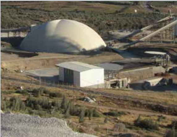
■ Additive Crusher and Additive Intake
