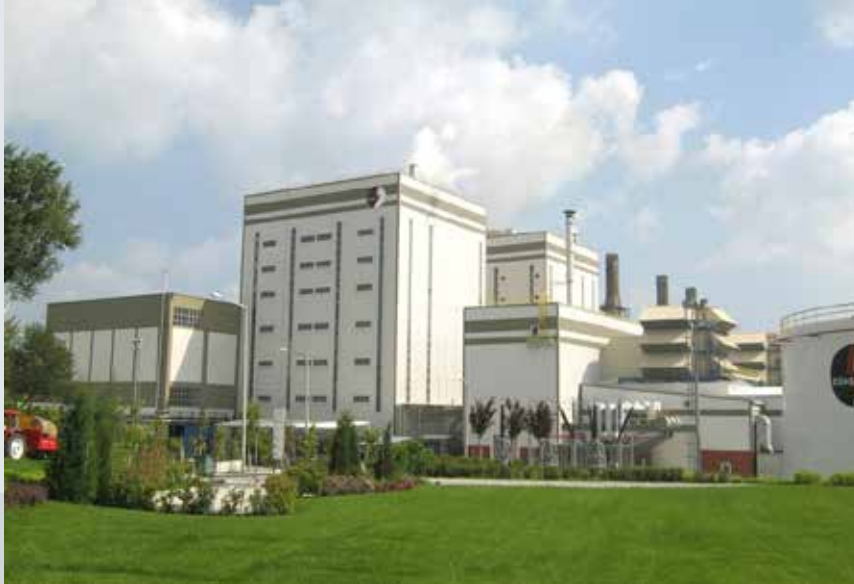
■ View of the New Ambarlı Power Plant
