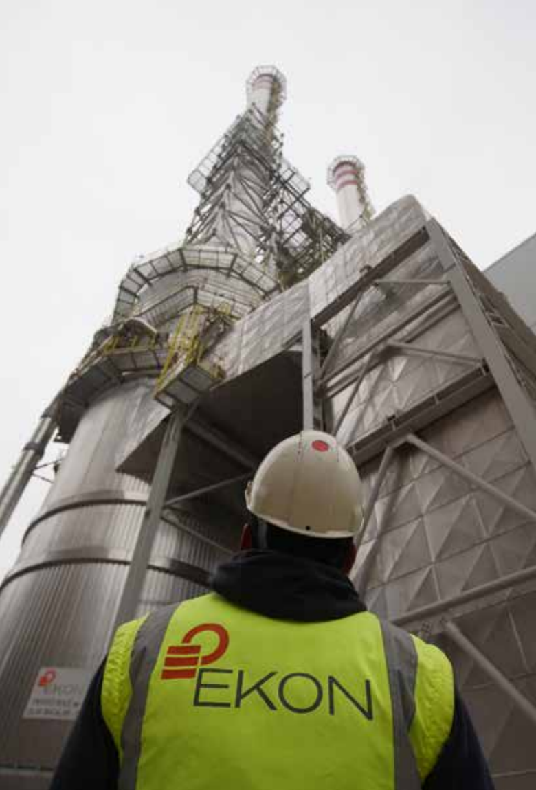
■ Wet Stack Steel Structure & +65.00 Level Platform
