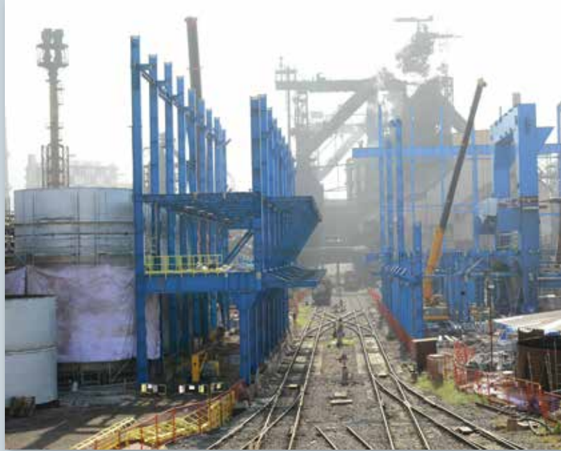
■ Hot Blast Stove and Casthouse Steel Structure
