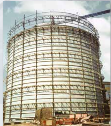
■ Construction Works at Outer Shell
