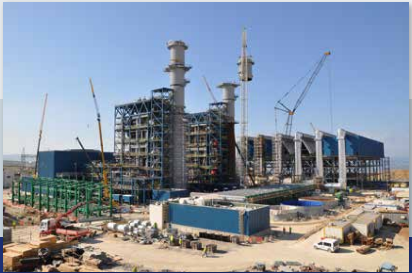
General View During Construction ■
