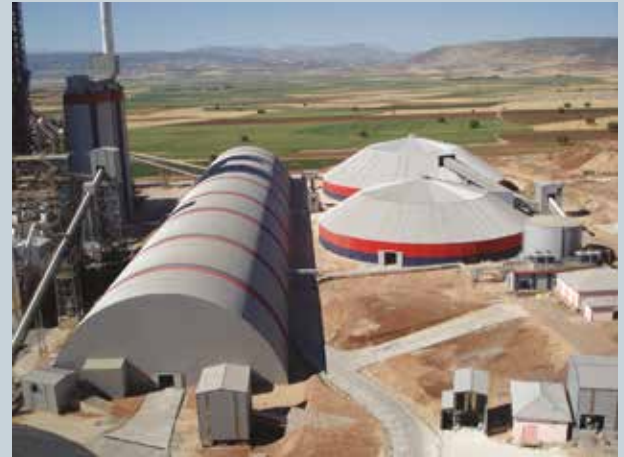
■ Circular Limestone and Longitudinal Shale Blending Bed
