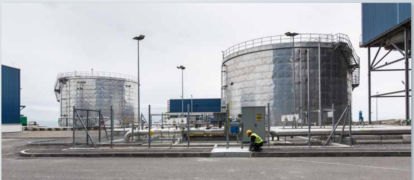
■ Raw Water Tank and Demi Water Tank
