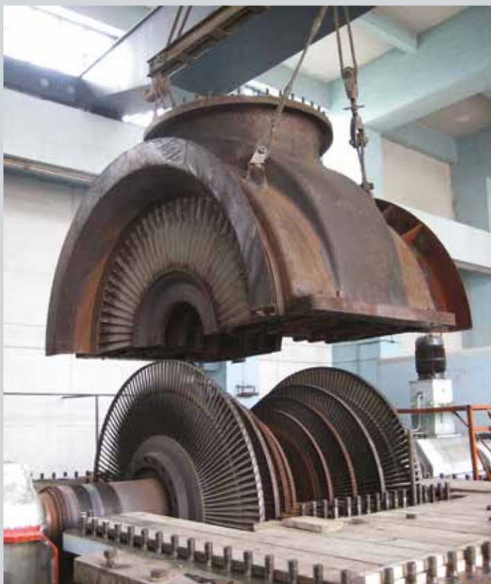
■ Steam Turbine Disassembly
