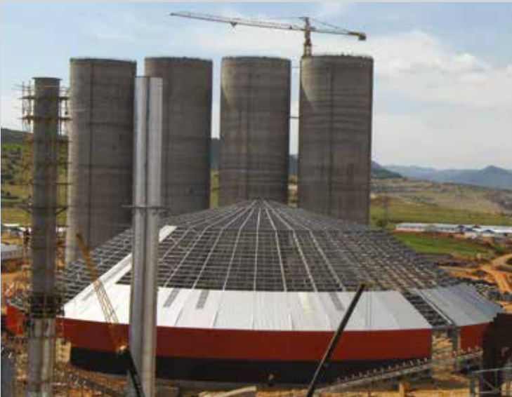
■ Circular Coal Mixing Bed and Cement Silos
